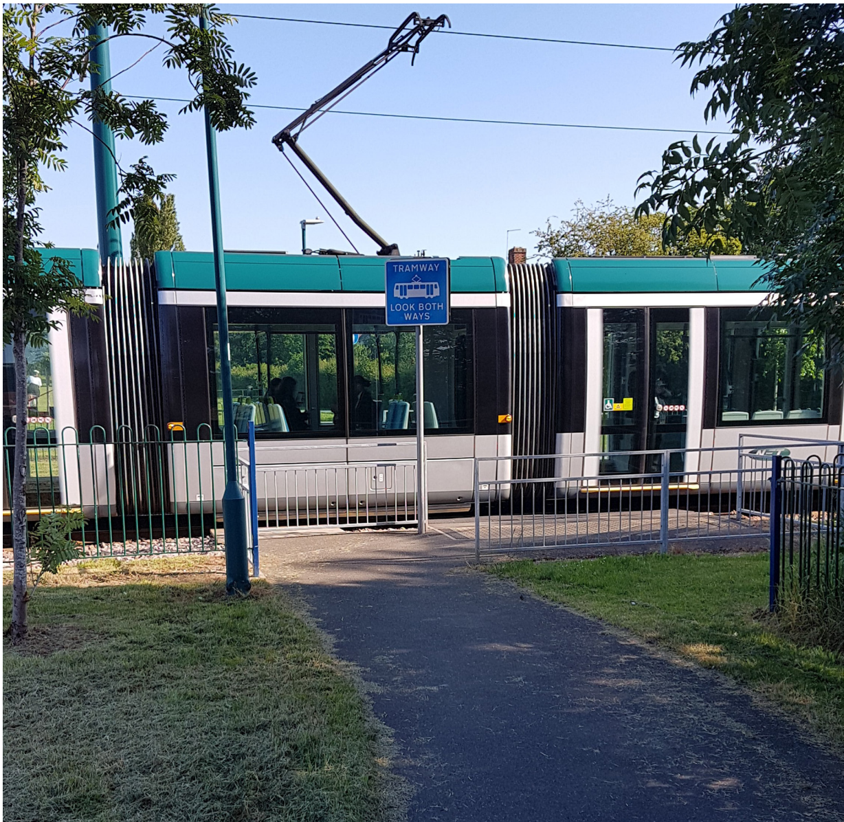
Figure 12: An example of chicane fencing on a footpath crossing on the Nottingham tram system. The tram in the picture is travelling on the closer of the two tracks from right to left.
