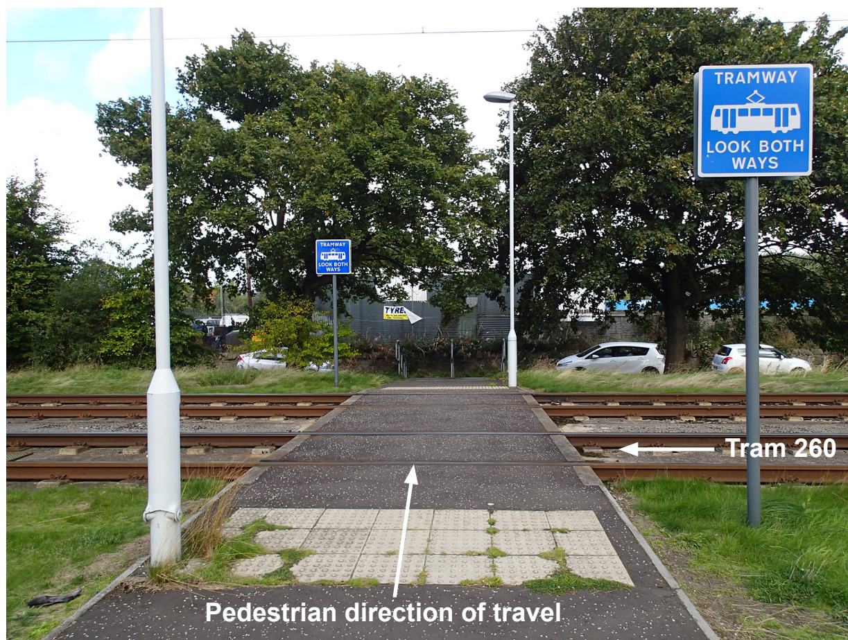
Figure 3: The approach to the footpath crossing looking north
