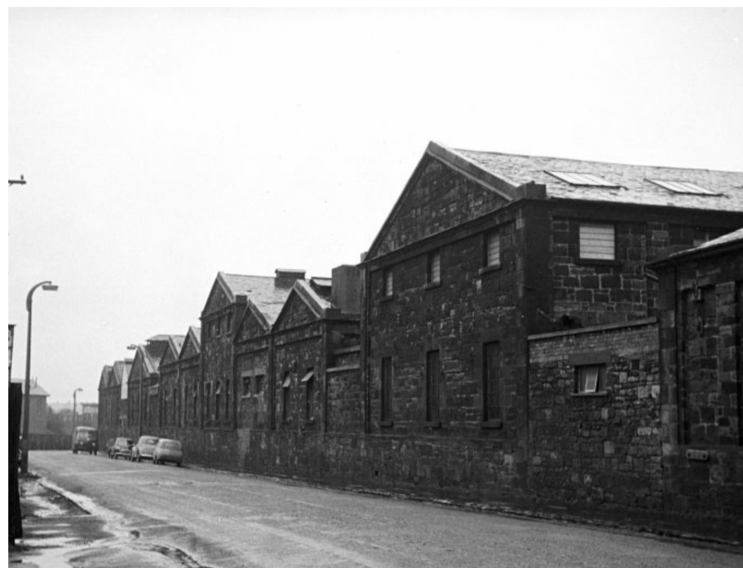
Exterior of St Margaret's Railway Workshops, Clockmill Road in 1966
