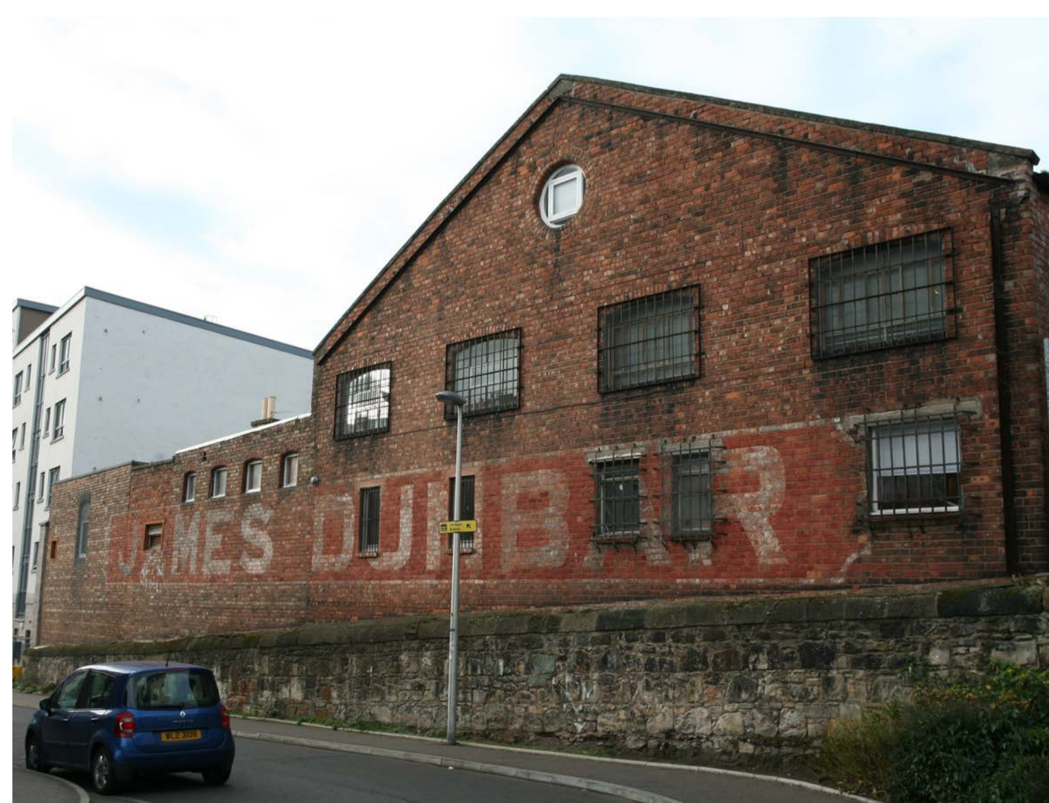
James Dunbar Ltd. former lemonade factory, Albion Road (constructed 1911)
