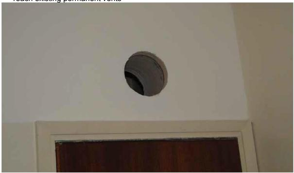
Figure 10 breach of fire-resisting enclosure
