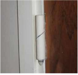
Figure 5 Rising butt hinge
